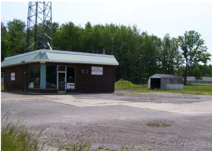
Northwest corner (right-of-way intersection) facing Southeast
